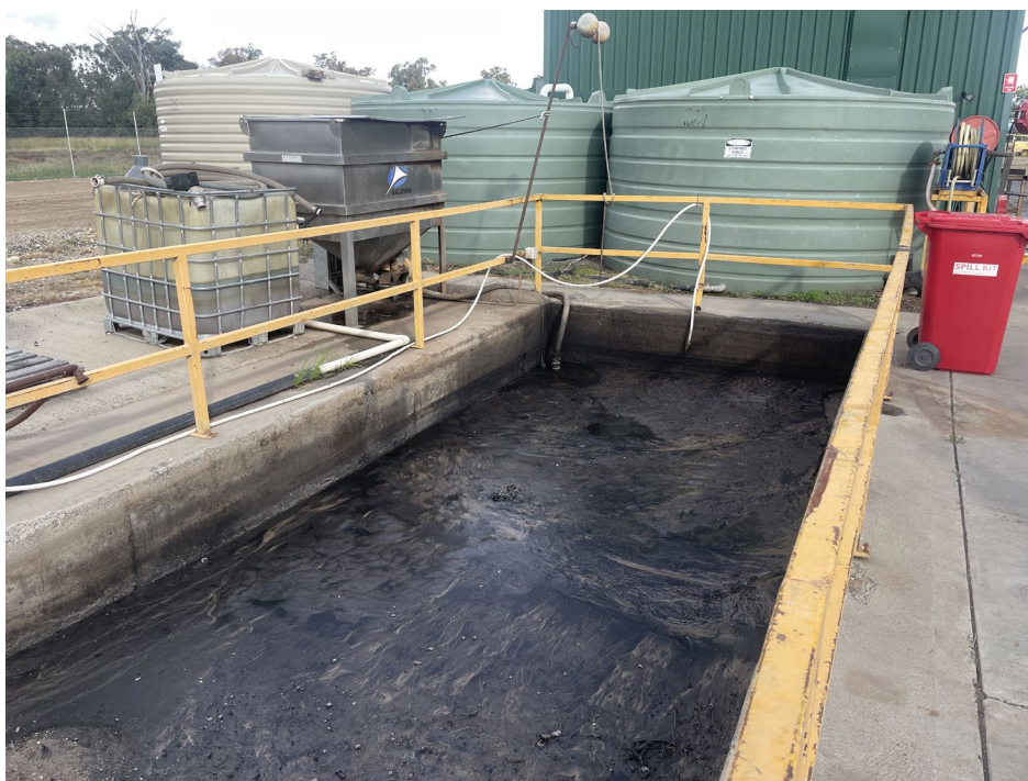
PHOTO 3 Mechanical workshop drainage sump
